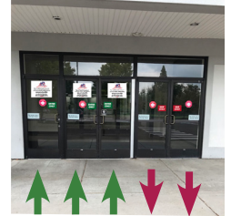
3 Doors to Entry. Do not Enter thru Exit
